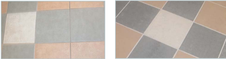
Restroom Floor Restoration Before & After
